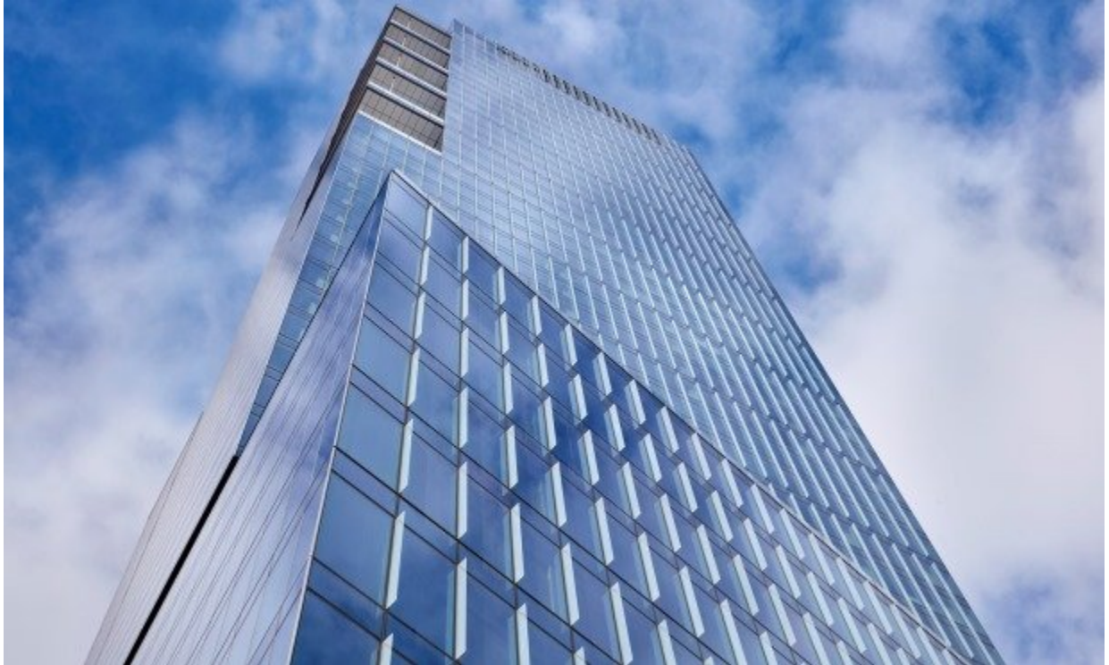
Large outdoor terraces are carved out to provide outdoor spaces or mini "parks in the sky" (credit: Tim Griffith).
